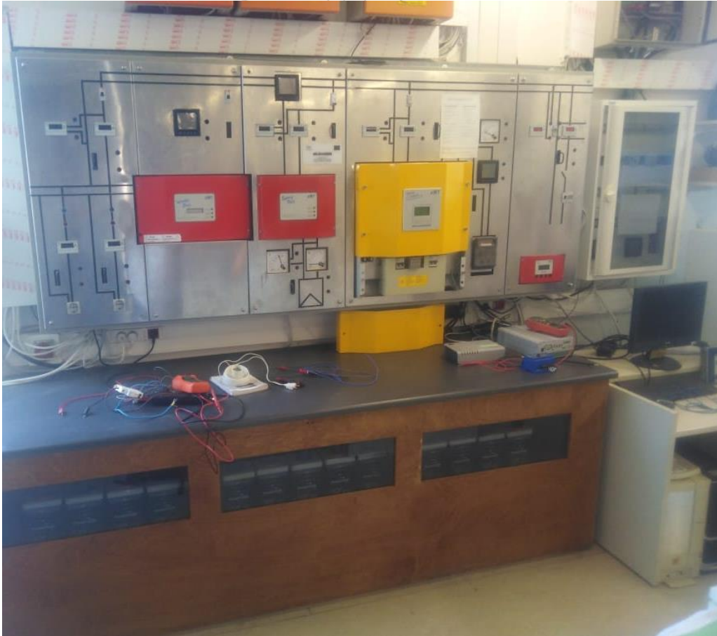
Fig4.The Low-voltage microgrid in the host lab
